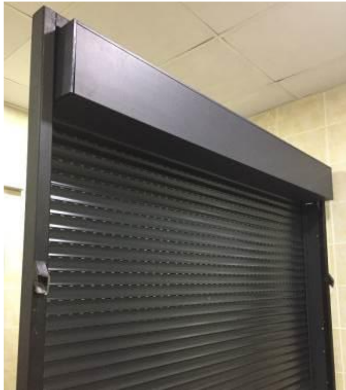
Photo 3. Shutter back top section
