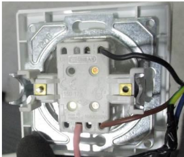
Photo 16. Rear surface of up-down move button
